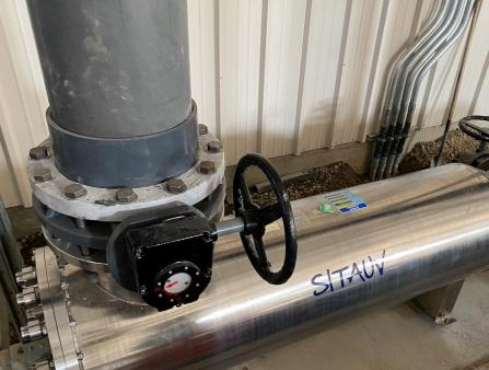
UV 440 Series is the industrial solution designed for flow rates between 50 and 3000 m<sup>3</sup>/h. Long life amalgam lamps are used in these units.
